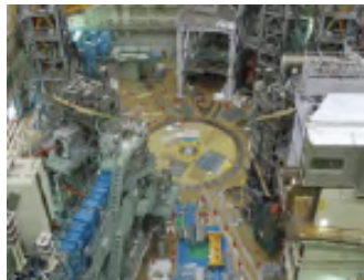
JT-60U Disassembly Completed in Oct. 2012 Cryostat Base
